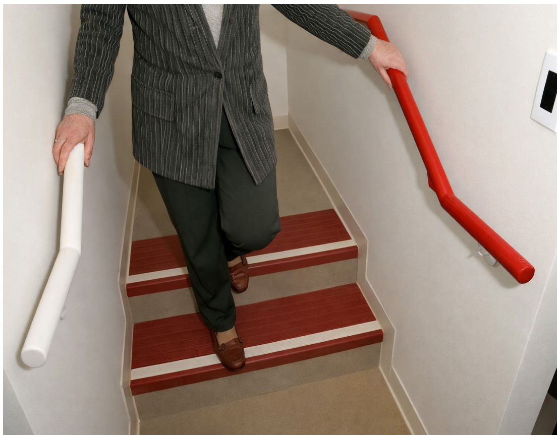
Fig. 10. Example of contrast use in indoor spaces
